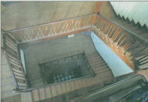
■ The restored Block 4 of Park Mansions.
